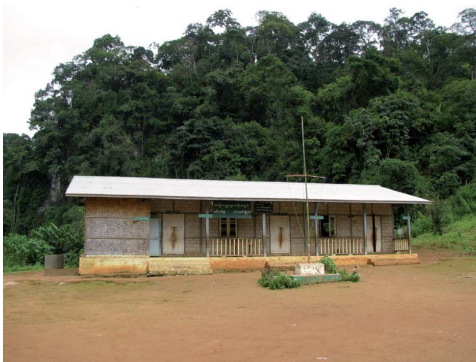
Primary school in a village. In spite of the simple building, the education provided in the schools is good.
